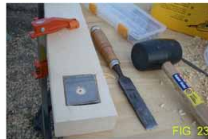
Figure 19- Fabricating 2" square stainless steel washers for final tie-off. Fig 20- Finished washers. Fig 21 Washers shown in final position with double nut. Fig 22- Mortise and hole for washer and nut shown. Fig 23. Cutting the mortice in board above to receive washer. Fig 24- Assistant shown applying epoxy to threads to lock double nuts in place.
