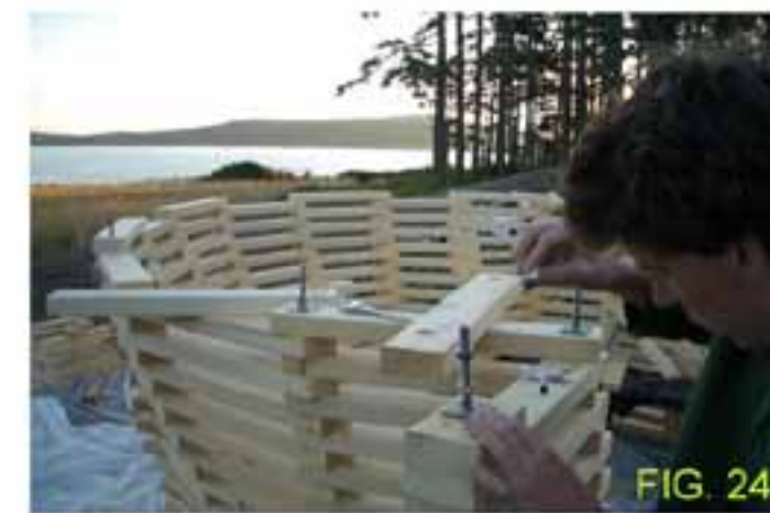
Figure 19- Fabricating 2" square stainless steel washers for final tie-off. Fig 20- Finished washers. Fig 21 Washers shown in final position with double nut. Fig 22- Mortise and hole for washer and nut shown. Fig 23. Cutting the mortice in board above to receive washer. Fig 24- Assistant shown applying epoxy to threads to lock double nuts in place.
