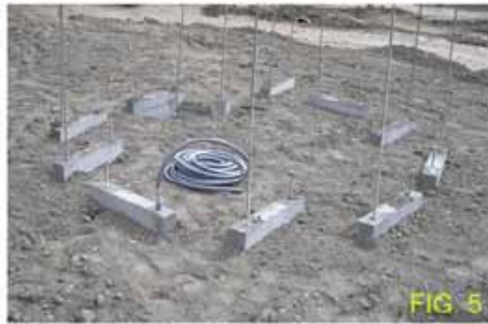
These images show the building of the footing for Daahoud. Figure 1 - Forming the slab. Figure 2- template used to transfer location of concrete 'teeth' that will support wood sculpture. Fig 3- Formwork for 'teeth' being located- note hole in center of slab for drainage. Fig 4- detail showing rebar, threaded rod, and conduit being located. Fig 5- completed footing covered with dirt. Note conduit for lighting, anchor bolts, and threaded rods for wind shear. Refer to Engineer's Report for details. Fig 6- Plastic sheeting covering the work area and carefully cut around each 'tooth'
