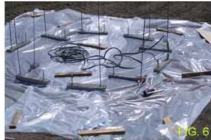
These images show the building of the footing for Daahoud. Figure 1 - Forming the slab. Figure 2- template used to transfer location of concrete 'teeth' that will support wood sculpture. Fig 3- Formwork for 'teeth' being located- note hole in center of slab for drainage. Fig 4- detail showing rebar, threaded rod, and conduit being located. Fig 5- completed footing covered with dirt. Note conduit for lighting, anchor bolts, and threaded rods for wind shear. Refer to Engineer's Report for details. Fig 6- Plastic sheeting covering the work area and carefully cut around each 'tooth'
