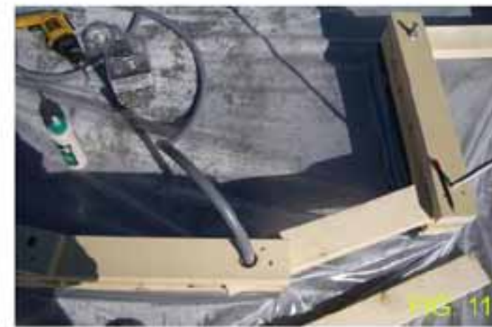
Figure 7- Drilling of the first board to fit over threaded tie down rods. All Lumber Alaskan Yellow Cedar, 2x4 x 2ft long. Fig 8- Placing of the first board. Fig 9- One and a half layers complete. Fig 10- Detail of threaded rod with first lumber layer bolted down and drilled out for nut and rod. Each layer glued down with Titebond III brand exterior wood glue, and additionally held by 2 #9 SS wood screws each end of each board. Fig 11- Location of conduit inside of boards. Fig 12- Three layers completed
