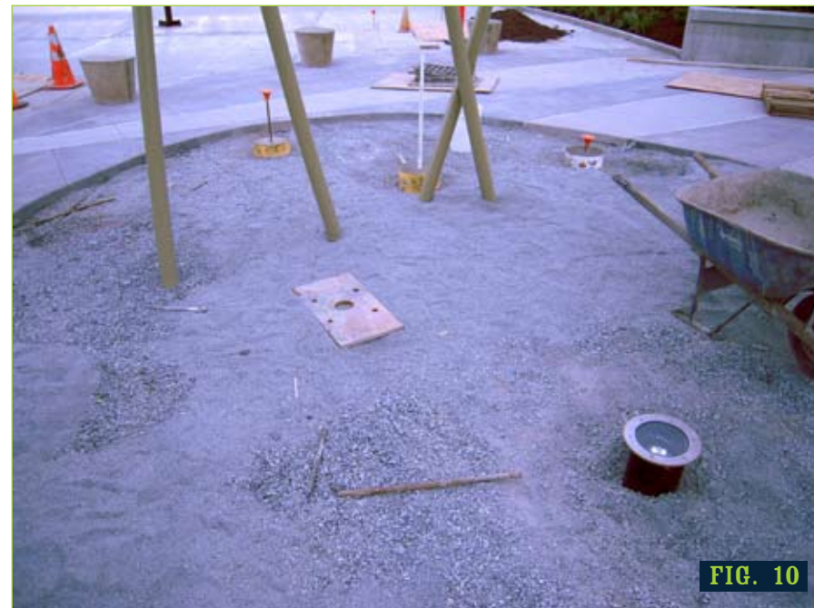
Figure 8- Internal view of completed sculpture, prior to removal of form work. Figure 9- The steel erectors, from Commercial Welding and Fabrication: L to R: Sean, Randy, Dave Figure 10- A view of the base, filled in with gravel. Note in ground light fixture in lower left
