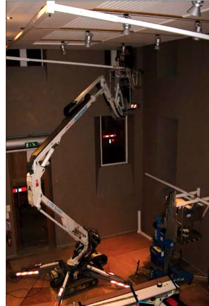
Rigging the steel armature into position.
